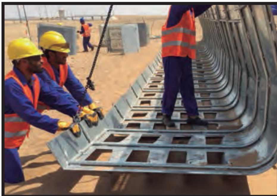
ASSEMBLY OF THE STRUCTURE
